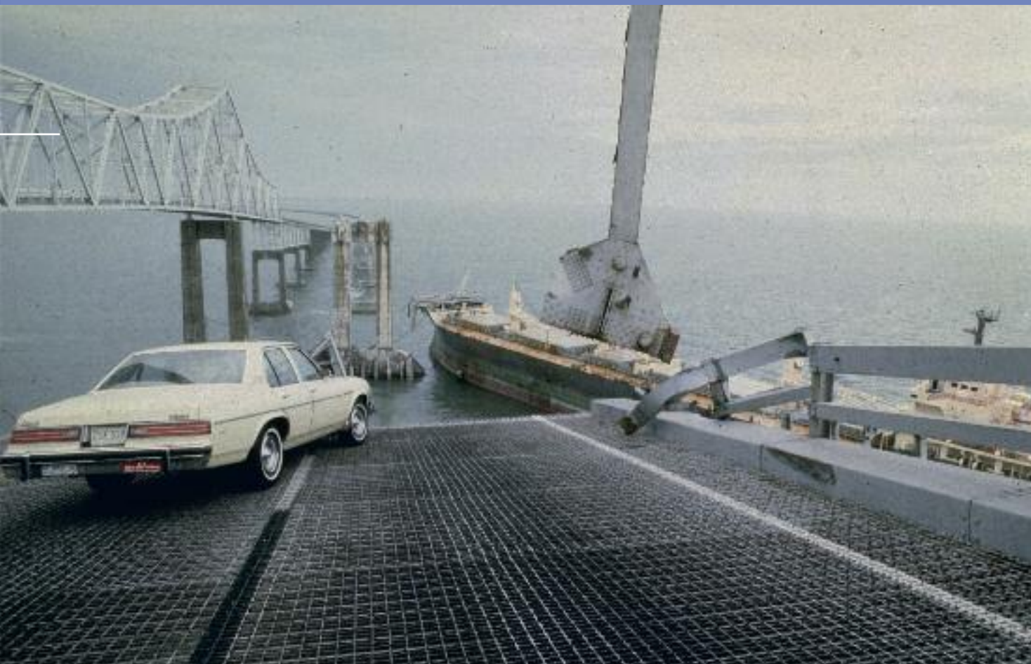
Entered Ships: The freighter Summit Venture struck the Skyway Bridge during bad weather in May 1980, causing the collapse of a large part of the span. Jackie Green / AP/Press Association Images
