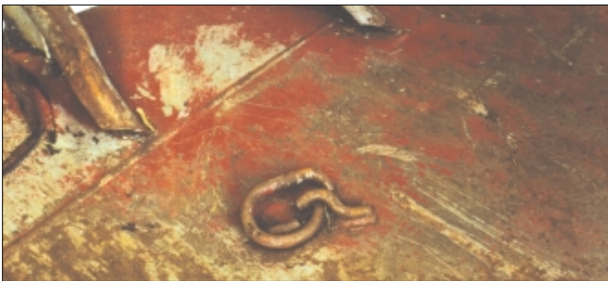
Proper training will help avoid failure of lashing points
